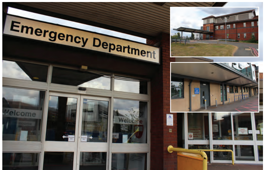
The survey focused on engineering plant and components in areas including the Accident and Emergency Department and Maternity Unit (top inset) Pharmacy, Pathology Department (bottom inset), ward blocks, and theatres - in all about two-thirds of the Walsall Manor Hospital’s retained estate.
